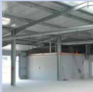
Industrial hall construction
